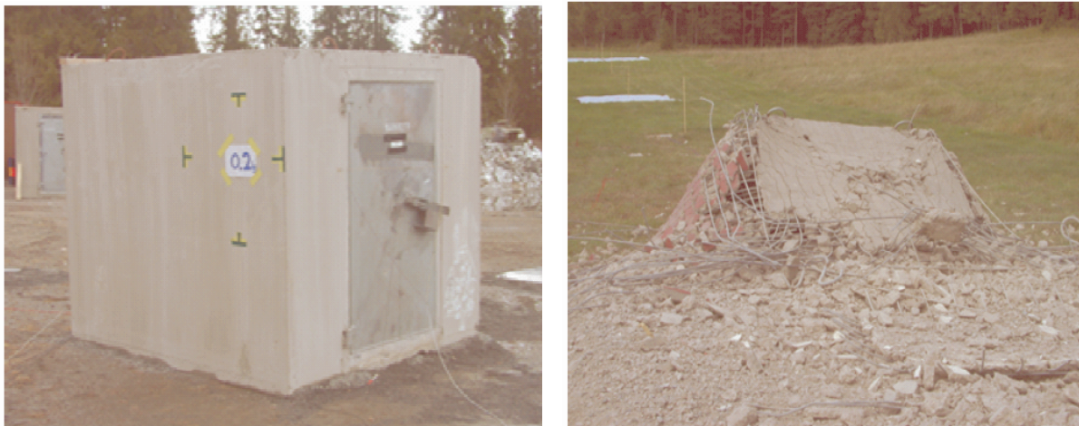
Fig. 3-8: Kasun storage building with an internal volume of 8 \text{ m}^3 (left). Result after detonation of 2 kg TNT (right). [Langberg 2004]
