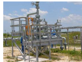
pics: KBB Underground Technologies GmbH
